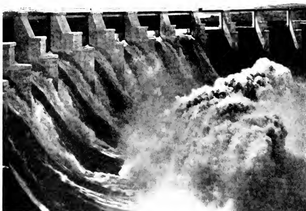
FIG. 5. GATUN SPILLWAY, WITH 7 OF 14 GATES OPEN, SHOWING EFFECT OF BAFFLE PIERS.
